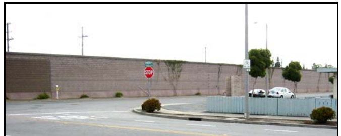
Site of the proposed pedestrian bridge. The ramp would rise along the sound wall, from left to right.
