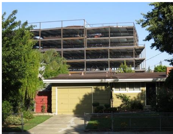
LinkedIn building construction as seen from Pine Ave.
